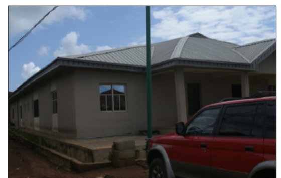
Renovation Of Onigogo Palace
