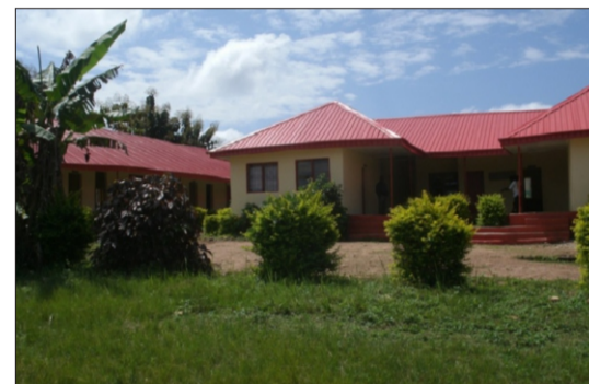
Renovation Of Ikosun Comprehensive High Schl.
