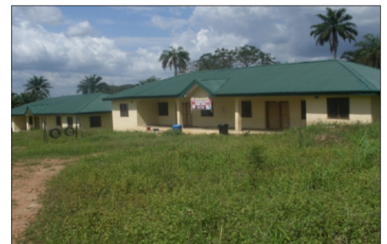
Construction Of 2 Maternity Wards in Igogo-Ekiti
