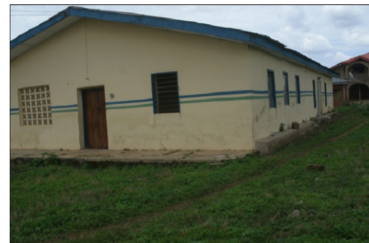
Renovation of Osun Police Station
