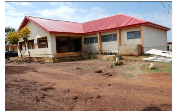
Renovation of General Hospital, Otun-Ekiti
