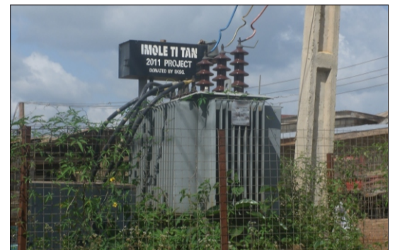
Installation of new transformer at Iro-Ekiti
