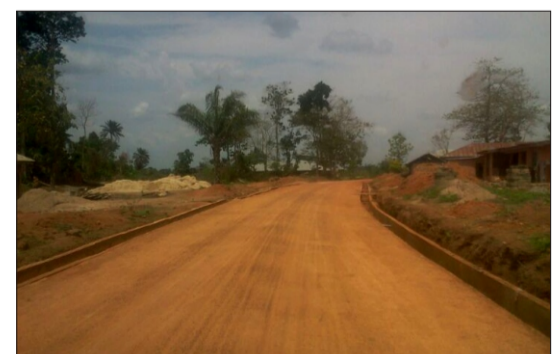
Ongoing 5km Road Epe
