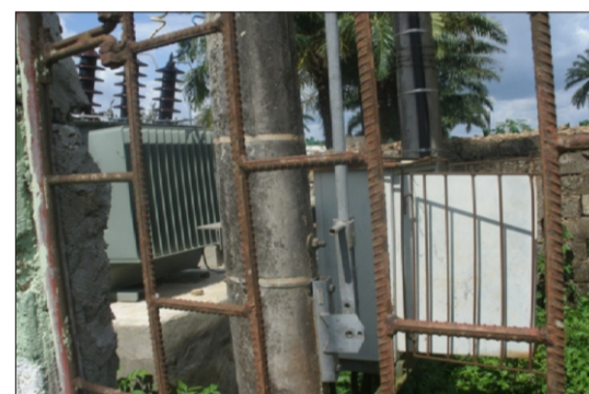
Installation of transformer
