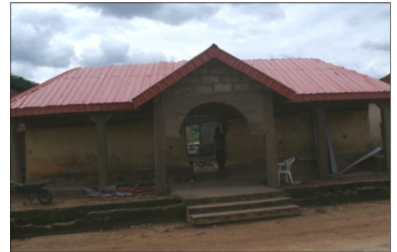
On-going renovation of the Aromiro Palace, Iro-Ekiti
