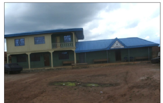
Renovation of Olosun Palace
