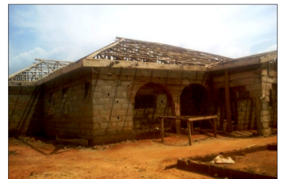
Ongoing Elepe's Palace, Epe
