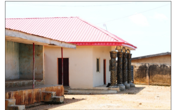
Renovation of King's palace, Erinmope
