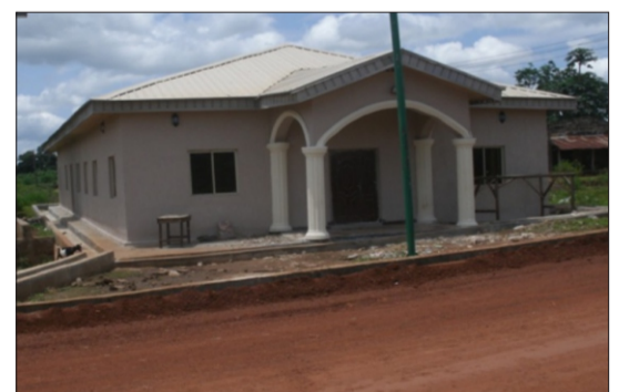
Renovation of Osan Town Hall
