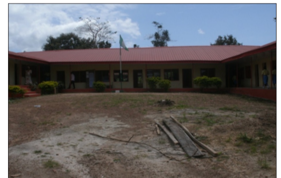
Renovation of Aaye-Oja High Sch.
