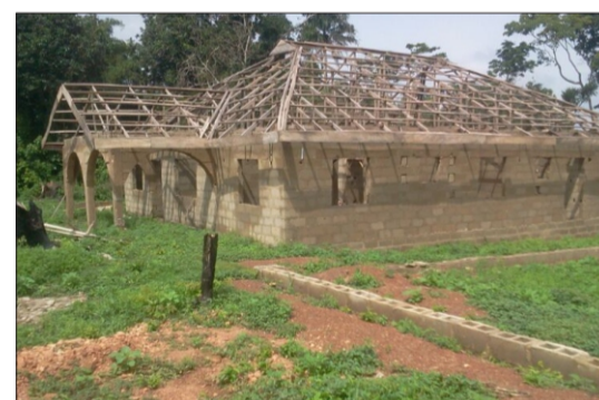
On-going construction of King's Palace, Ira-Ekiti
