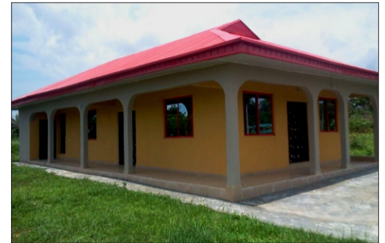
Completed Town Hall Irare
