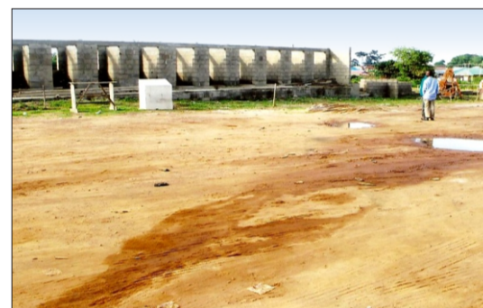
On-going construction of trailer park at Omuo Oke-Ekiti
