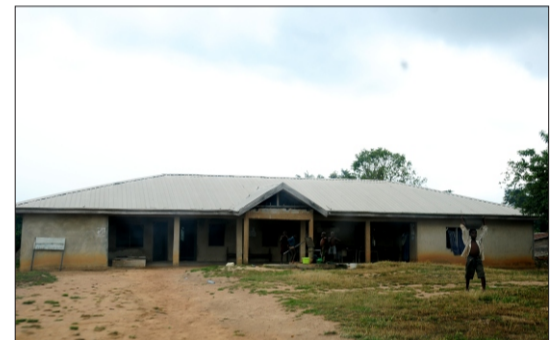
On-going construction of Basic Health Centre, Ikun Araromi-Ekiti,
