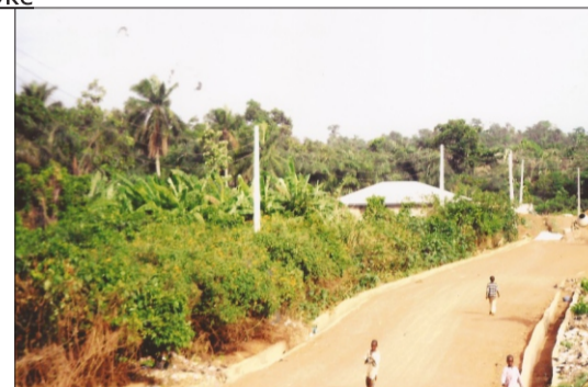
Construction of 300m Araromi Oke- Igbagun road.
