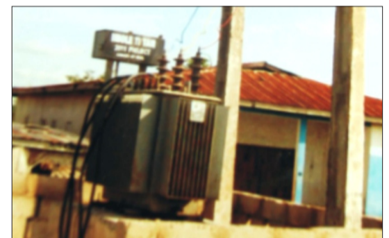
Installation of 3 Units of 300KVA Transformer.
