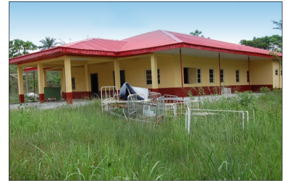
Renovation of General Hospital, Omuo - Ekiti
