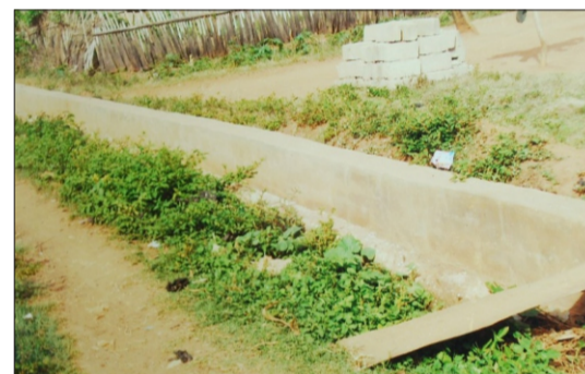
50m drainage construction at Odo Oyi St, Araromi-Oke.
