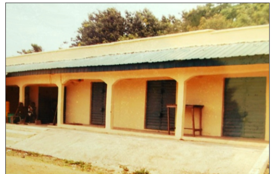
Construction of six rooms lock-up shop stalls at Adumari Street.
