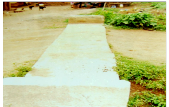
Construction of Culverts at Ilasa.
