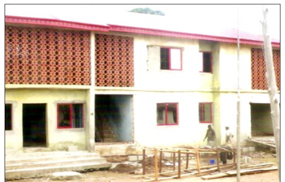
On-going renovation of Oba's palace, Ilasa
