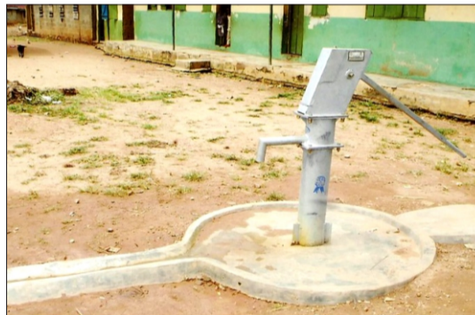
Provision of Hand pump borehole at St. Paul's Primary School.
