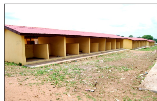
Renovation of Obada Market, Emure.
