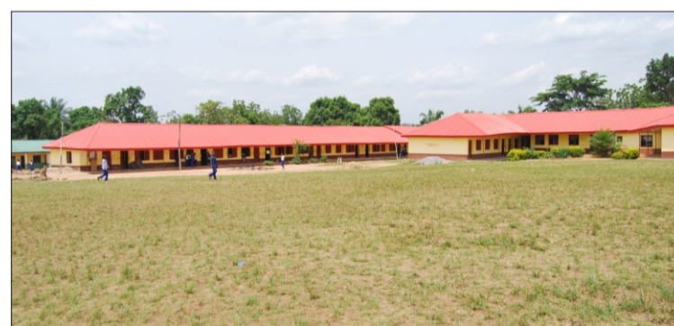
Renovation of 2 Blocks Of Classrooms at Ijaloke Gramm. School, Emure-Ekiti
