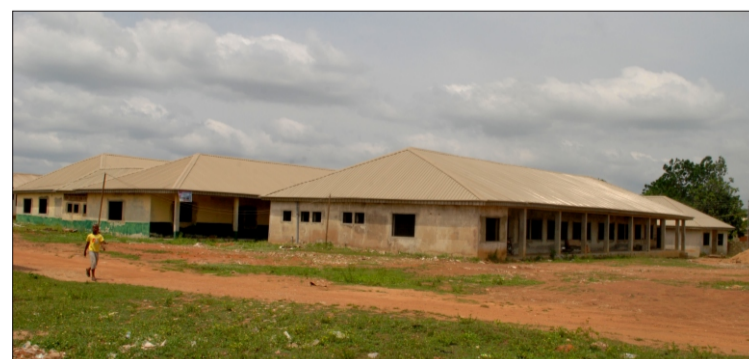
Renovation of 4 Blocks at Emure General Hosp.
