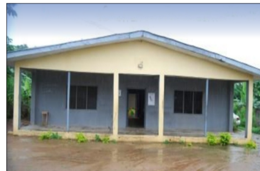
Renovation of Health Centre at Afolu, Ise-Ekiti
