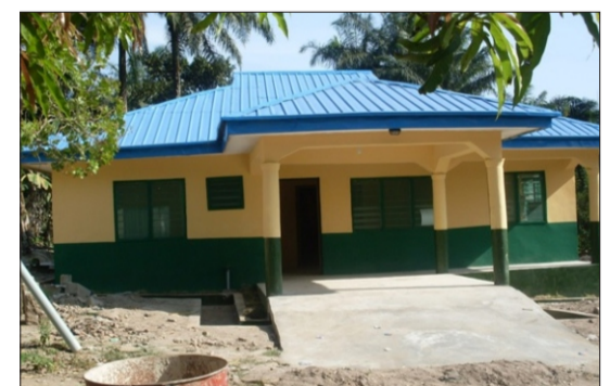
Construction Of A Basic Health Centre - Ise
