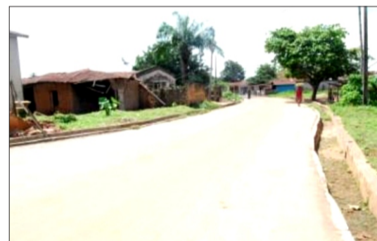
Construction of road at Bolorunduro Street, Orun-Ekiti
