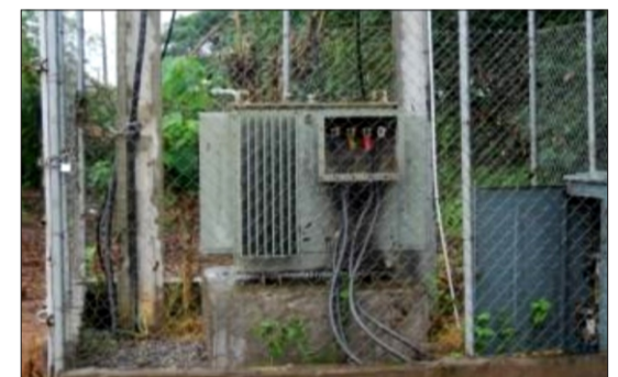
Installation of transformer at Oke-Odi Street, Ise-Ekiti
