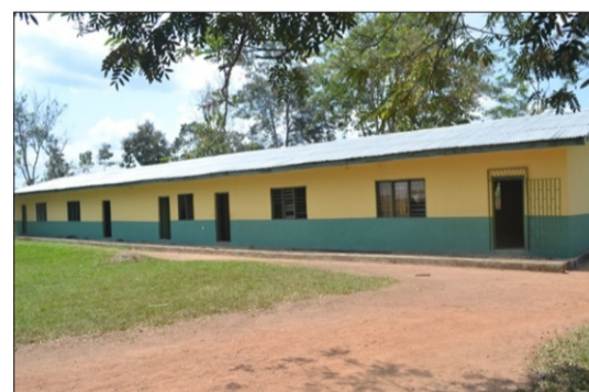
Renovation Of Science Laboratory, Orun-Ekiti
