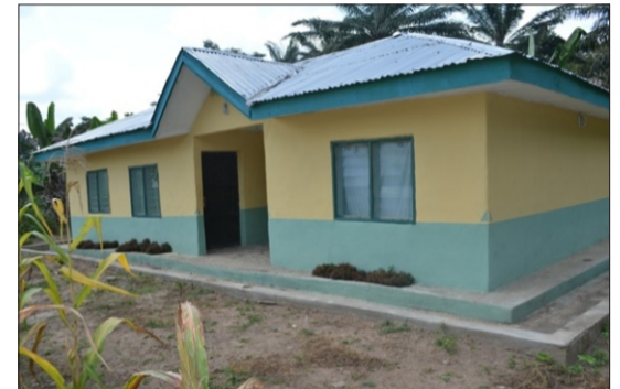
Completion Of Doctors' Staff Quarters, Ise-Ekiti
