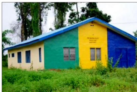
Completion of Police Post at Orun-Ekiti
