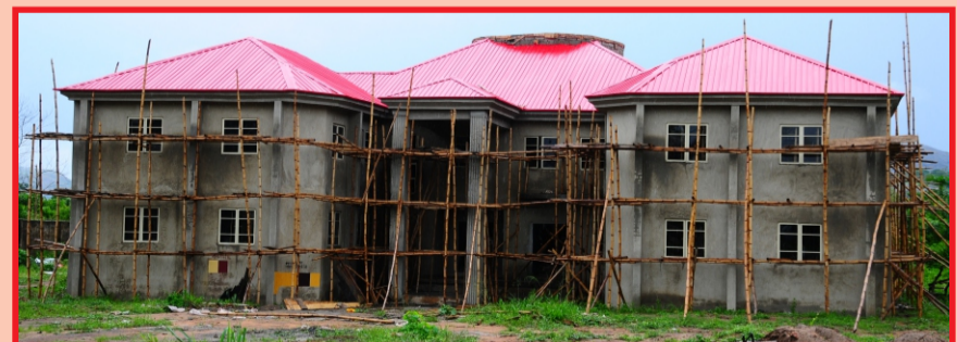
Administrative Building (under construction)
