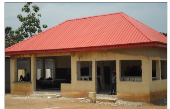
Renovation of General Hospital, Aramoko
