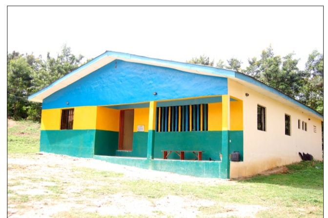
Construction Of Police Station At Okemesi
