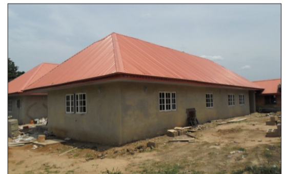
On-going renovation of the King's palace, Aramoko
