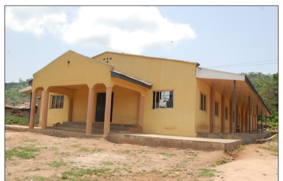
Completion Of Commercial Viewing Centre At Ido Ile
