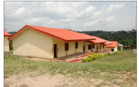
Renovation Of Edu High Schl, Erio-Ekiti
