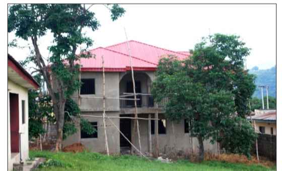
On-going construction of Oba's palace
