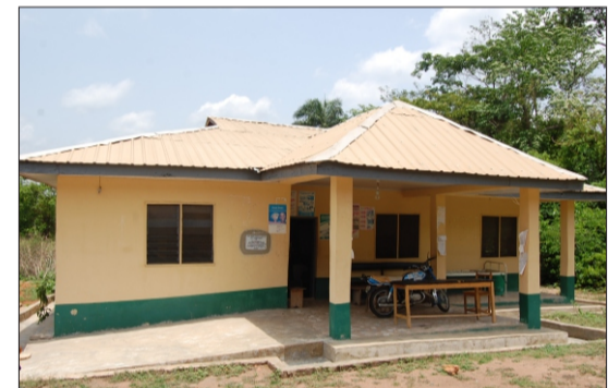
Construction Of Basic Health Centre At Ido Ile
