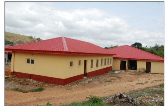
Renovation Of General Hospital At Okemesi
