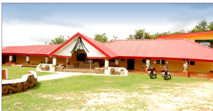
Renovation Of Owa Ooye Palace, Okemesi
