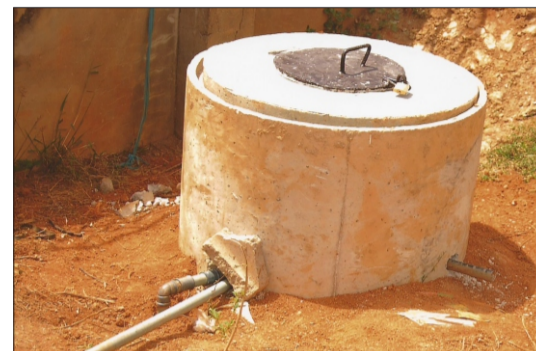
Hand dug well at Prof. Taylor street. Eejiyan.
