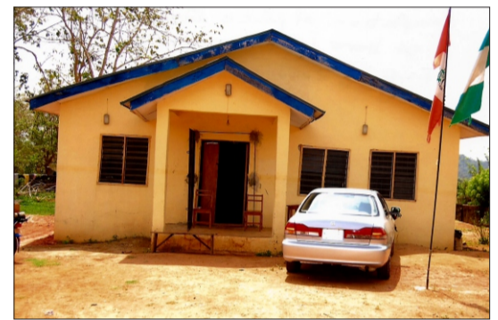
Completion of Police Station, Igbamitoto, Ijero.
