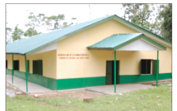
Renovation Of Examination Hall, Ikoru
