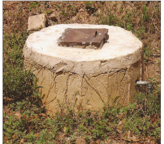
Construction of Handdug well, Temidire.
