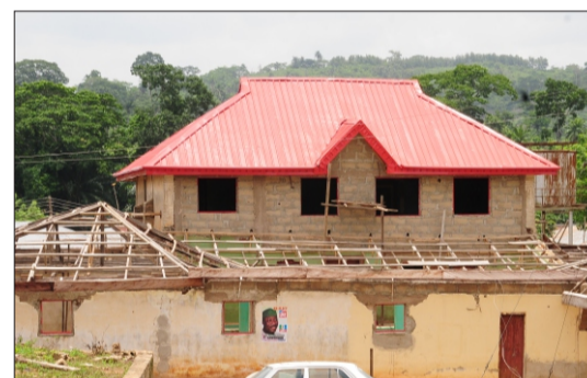
Ongoing renovation of Obas Palace, Epe-Ekiti.
