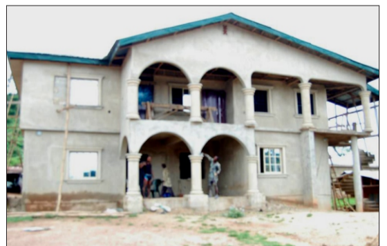
Construction of New Oba's Palace at Odo-Owa.
