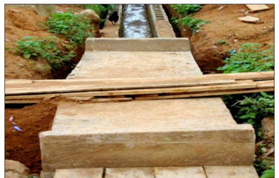
Ilukuno Construction of a Box & Ring Culvert
