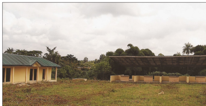
Construction of Modern Abattoir, Ijero.
