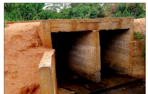
Double box culvert at Ara.
