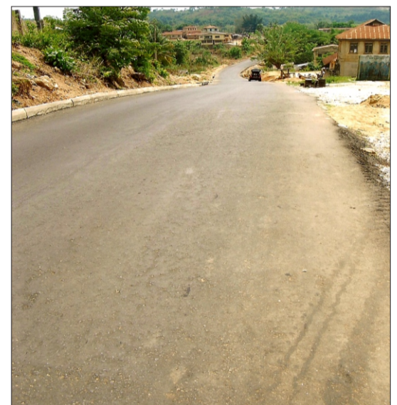
5km road project at Ifakin Street, Ijero
