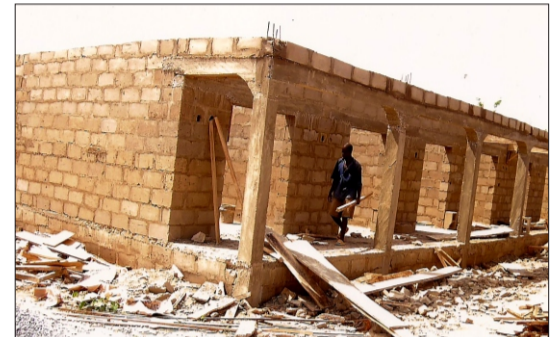
Construction of modern market at Igbamitoto, Ijero.
