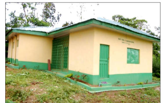
Construction Of Craft Skill Acquisition Center At Ikoru-ekiti
