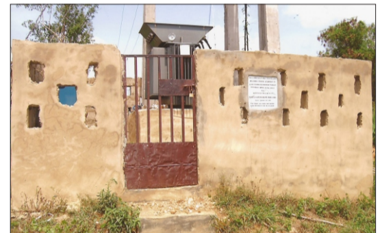
Installation of 300kva transformer, Ijero
