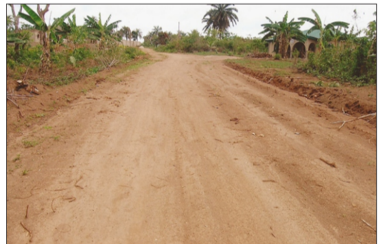
Grading of Roads, Ilukuno.
