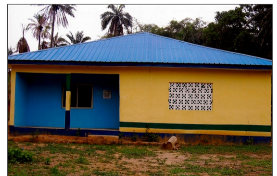
Construction of Police Station, Ara-Ekiti
