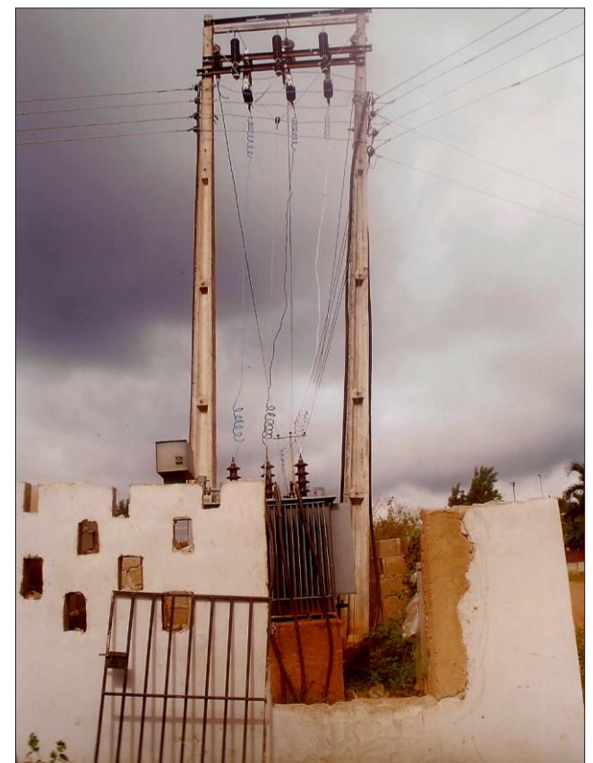
Purchase & Installation of Transformer, Ipoti.
