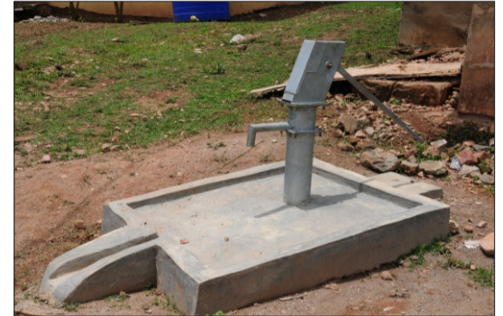
Borehole at St. Mary Cath. Pry Schl, Araromi-Ekiti.
