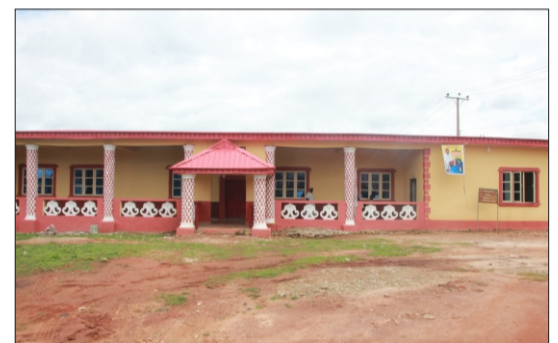
Construction Of Iloro Civic Centre, Iloro.
