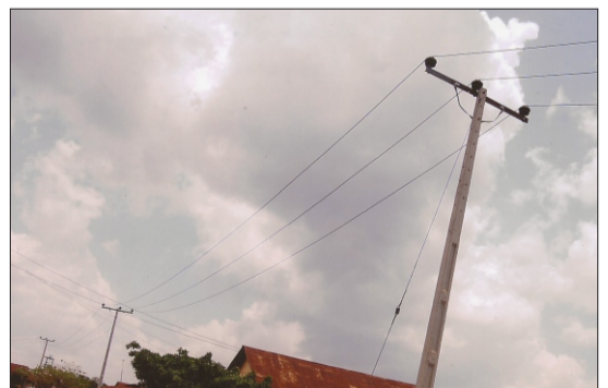
Electricity extension at Ayegunle high school, Ayegunle.
