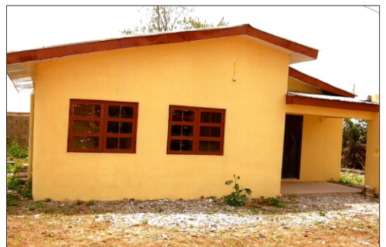
Renovation of Peace Corps building, Ogbamitoto, Ijero.
