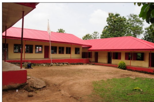
School renovation at Ekameta Com. High Schl, Epe-Ekiti.
