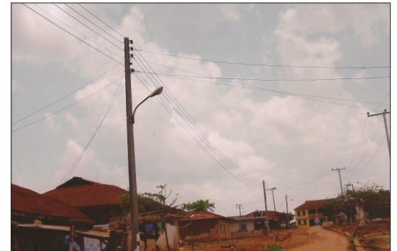
Electricity extension at Osere str. Ipoti.
