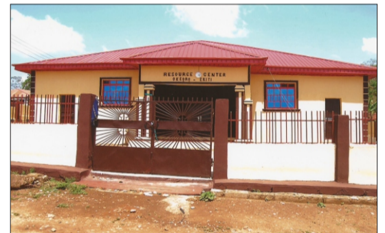
Construction of Resource Centre, Oke-Oro
