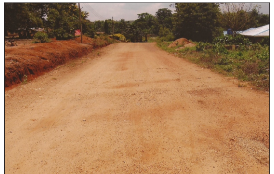
Road Grading at Ayegunle
